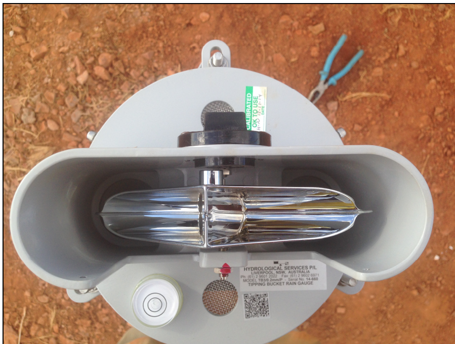
Figure 4 – Tipping Bucket Rain Gauge with catch removed during installation
